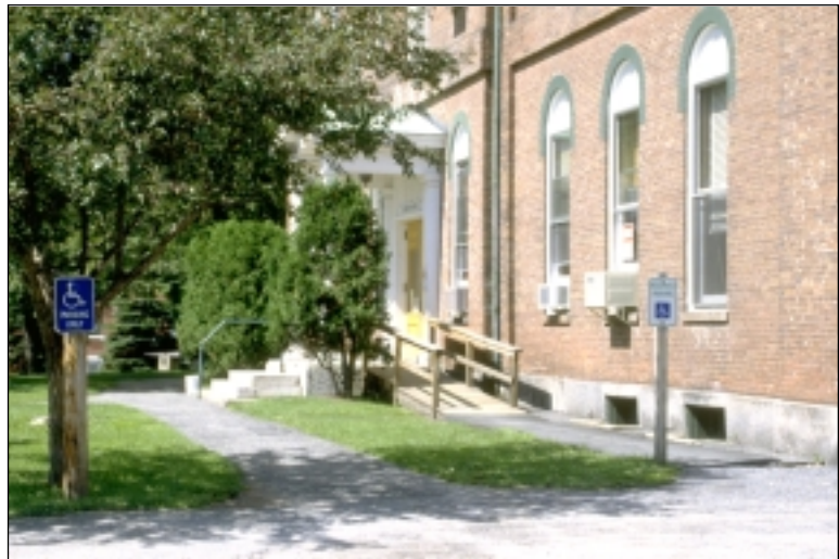
A ramp was installed to provide access to the city activities conducted in this facility.
