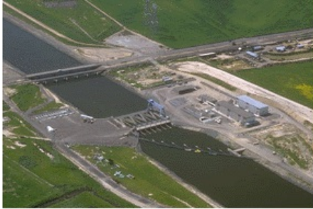
Skinner Delta Fish Protective Facility in Byron, California
