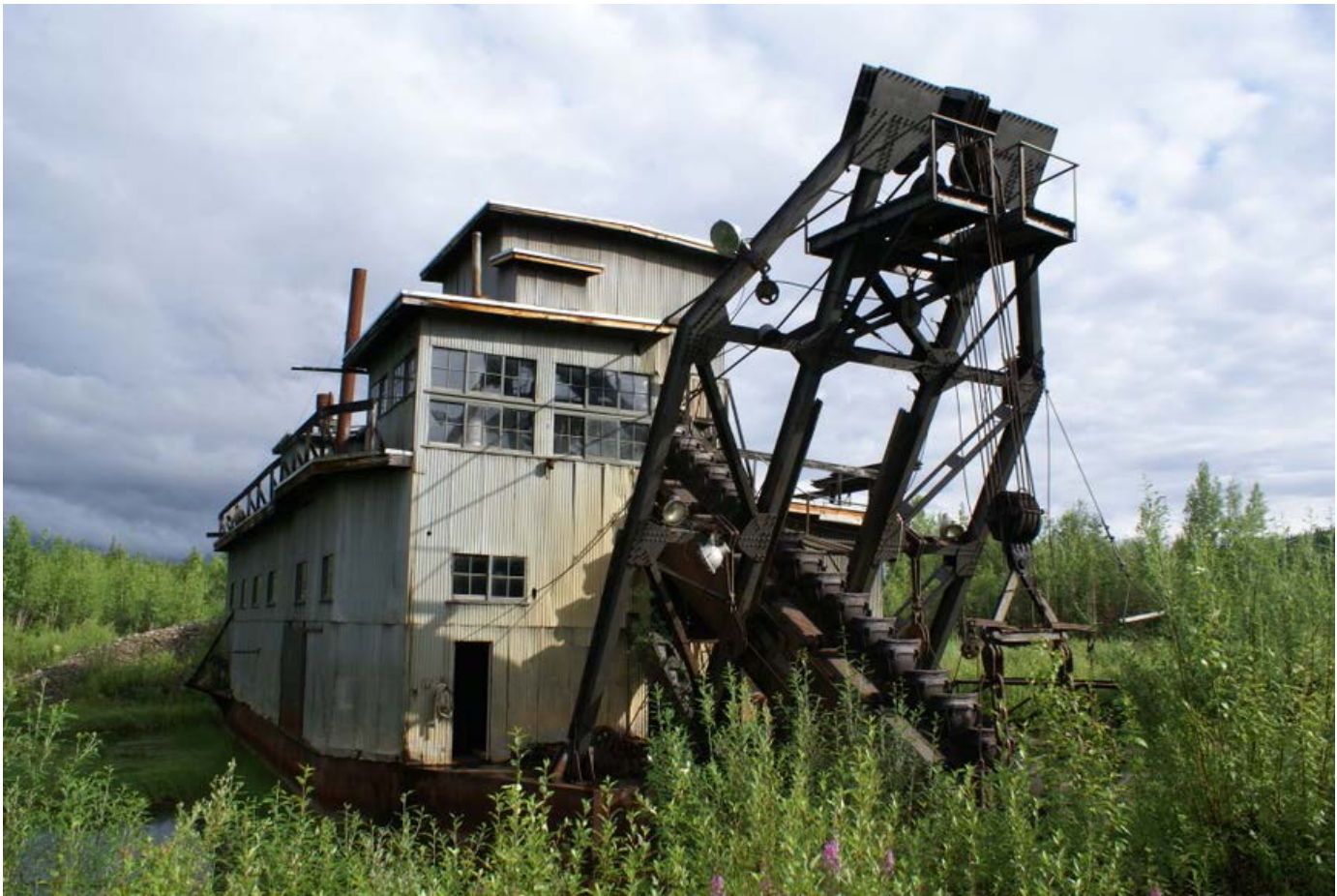
The Coal Creek dredge.
