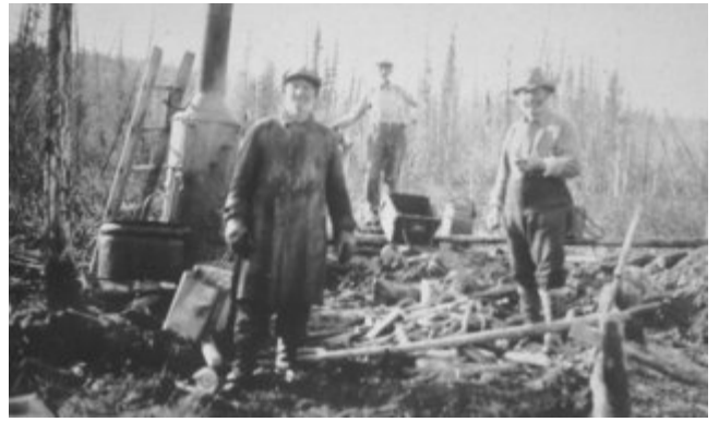
Placer miners using a small steam boiler and drift mining techniques on the Charley River, 1930s.
