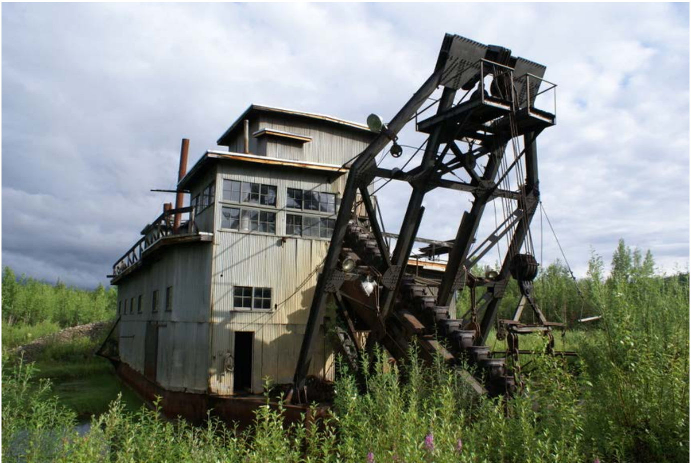
The Coal Creek dredge.
