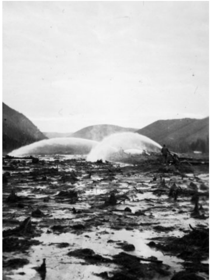
Using hydraulic "giants" to thaw frozen ground, ca. 1936.
