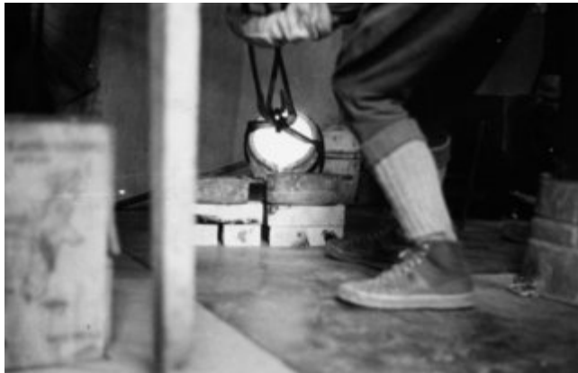
Turning molten Coal Creek gold into bars, 1936.
