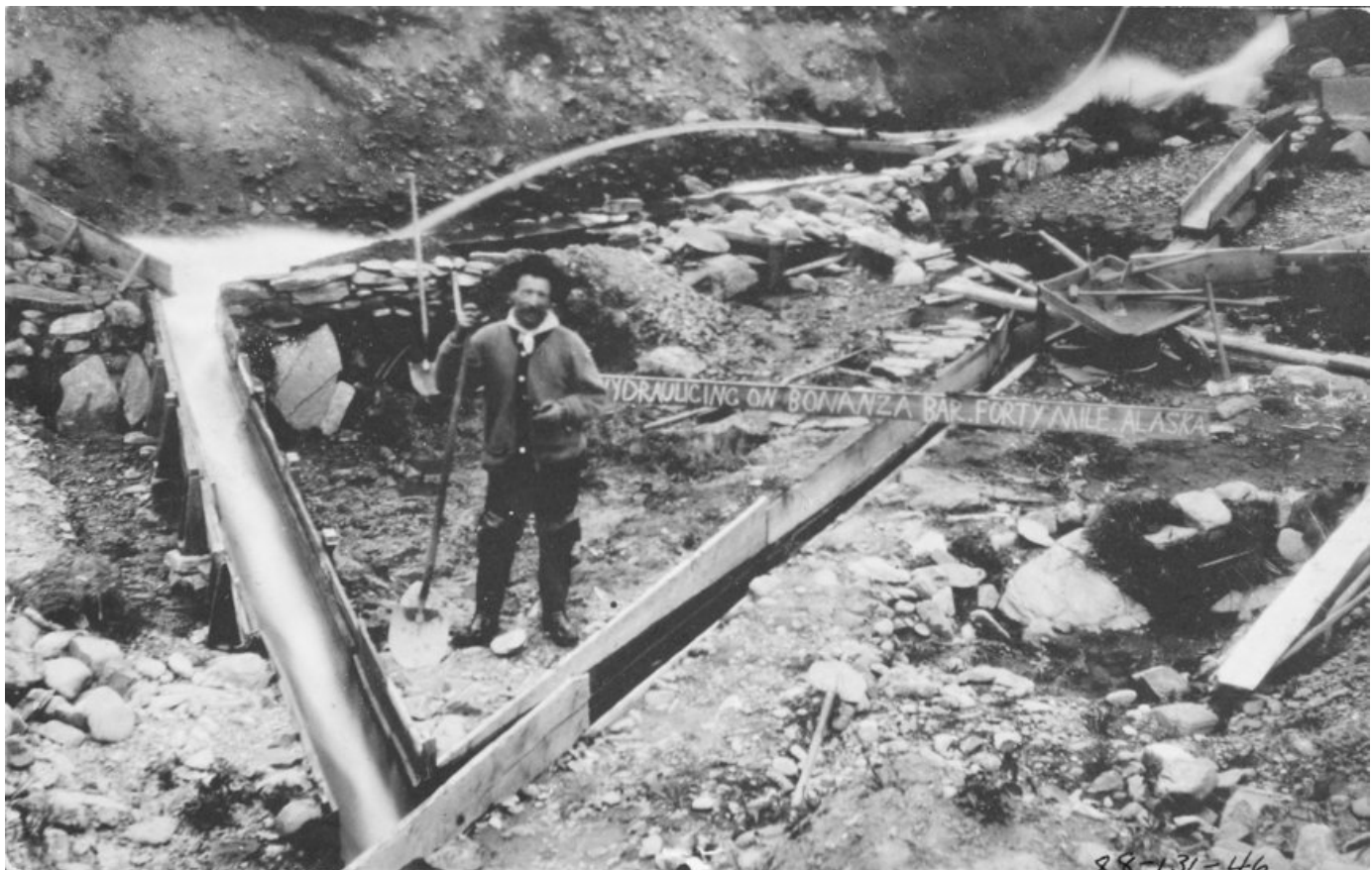
Hydraulicking with sluices boxes near the Fortymile River, ca. 1915.
