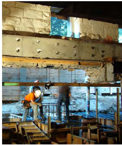
Crews working on the Pioneer Courthouse seismic retrofit.
