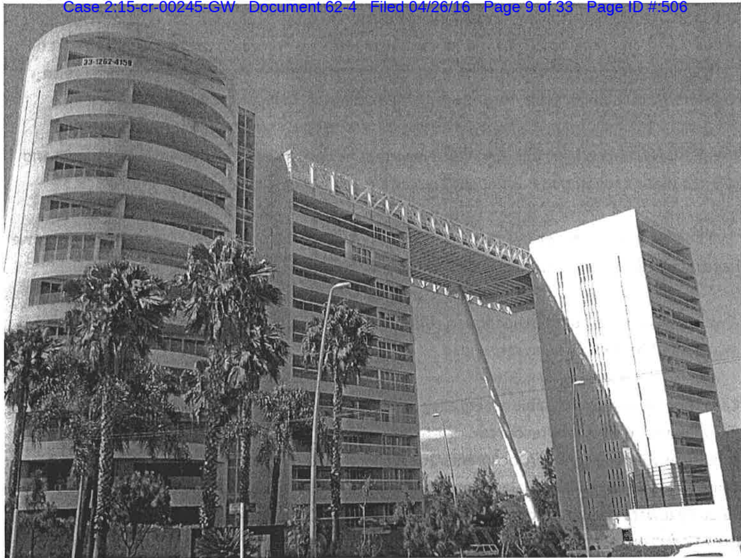
Two 12-story towers in Guadalajara allegedly linked to drug lord Rafael Caro Quintero. (Photo by Duncan Tucker)
